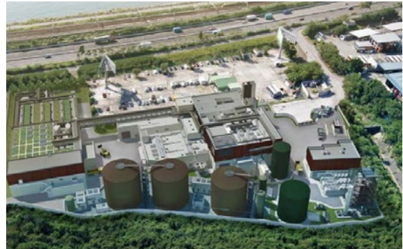
Hong Kong's Organic Resources Recovery Centre
