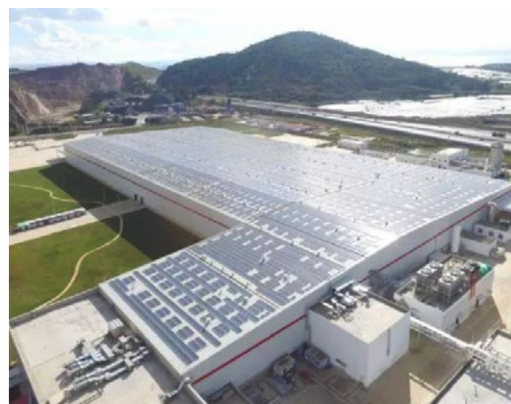
LEED Platinum certified bottling plant in Yunnan, Mainland China
